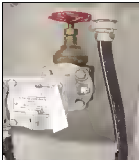
Figure 32 – Photograph of a Sudden Pressure Relay.
